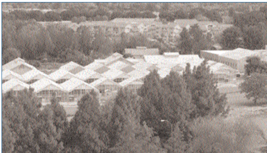
Can you locate the Student Farm Field House -- originally known as the Truck Crops Bulb House -- among the new plant sciences facilities?
